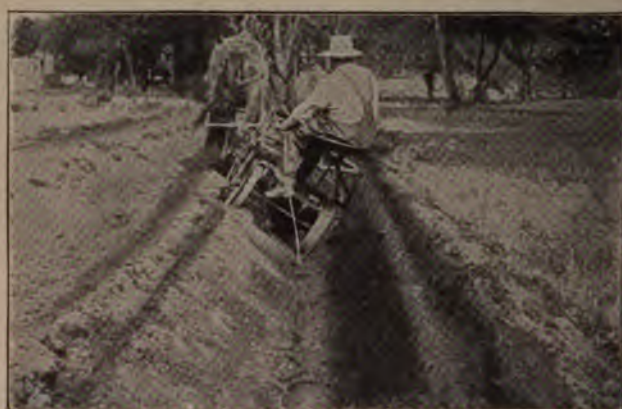
Two-wheel Grader Excavating Ditch.
